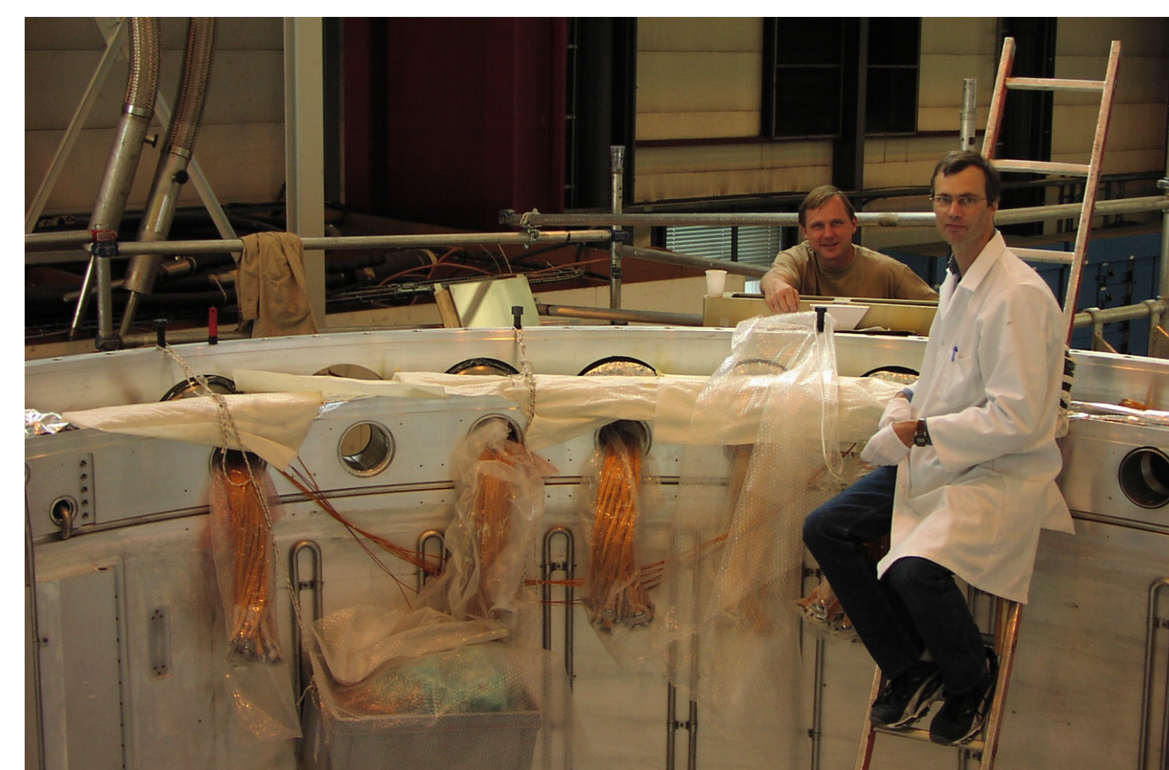
Paul Birney (TRIUMF) and Ken Sexton (BNL) at CERN after the installation of pedestals and warm cables. September 2003.
