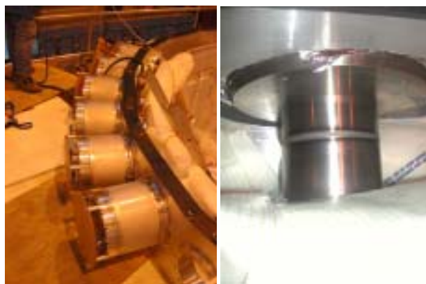
Fig. 4. First six feedthrough units installed on the first endcap cryostat (December 2002) and a close-up on one of the welds. Photos by Aboud Falou, Orsay.
