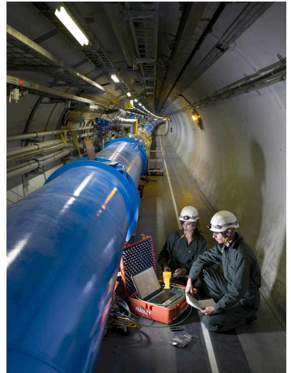
LHC magnets operate at 1.9 K 1232 dipoles (8.4 T, 34 t) 392 quadrupoles
